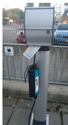
Fig 4 - Mode 2 ladeboks – oppheng mangler
